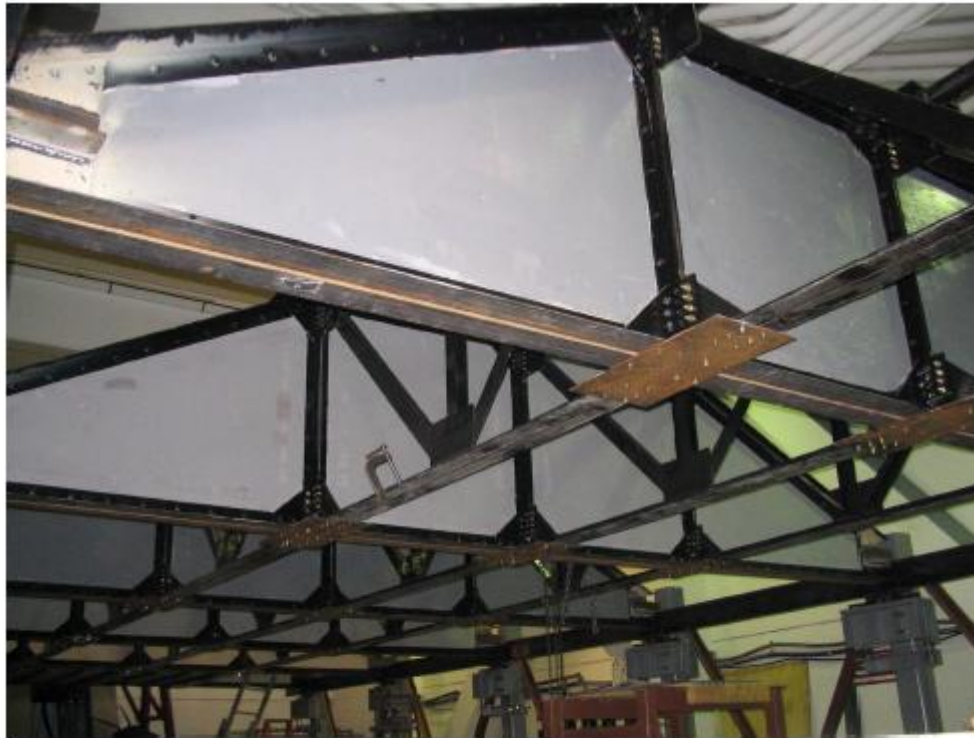
Figure 14: The Ceiling Structure
